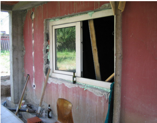
The windows you sent are being installed.
