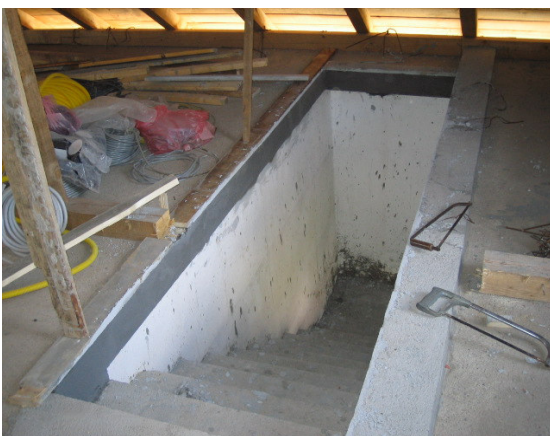
The ring around the balcony stairs is finished and the fence with a small door will be made for safety reasons. More windows in the guest room with walls ready for painting. This job will be left for FMWT.
