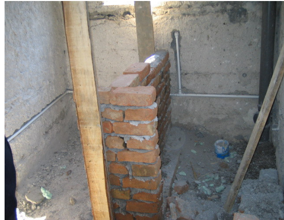
The inside toilets are being built.
